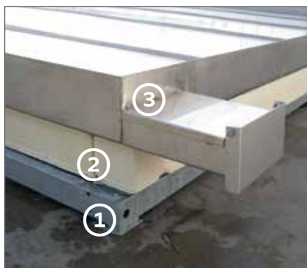
1 supporting frame 2 insulation panels 3 tub with drainage
